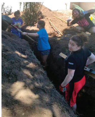
We dug a trench around a church to prevent water from getting into the basement and flooding it.
