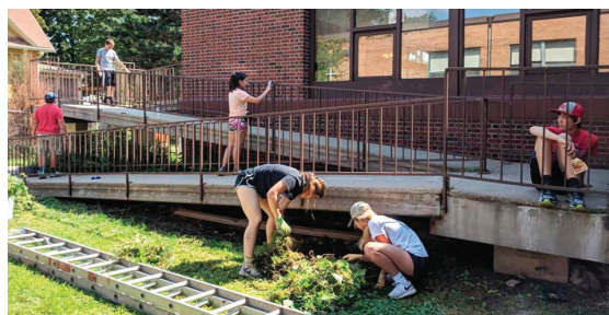
We dug a trench around a church to prevent water from getting into the basement and flooding it.
