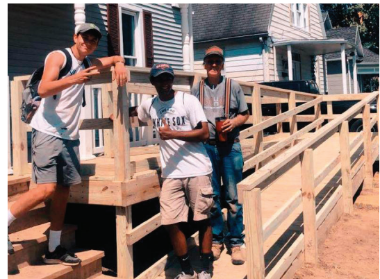
Built a wheelchair ramp at a residence.
